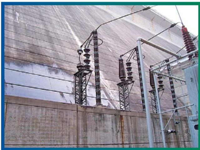
**THE UNIT 1 TRANSFORMER CABLE POTHEAD WAS SEVERELY DAMAGED IN A SEPTEMBER 6, 2006, EXPLOSION. SOUTHWESTERN IS WORKING WITH ITS CUSTOMERS AND THE CORPS TO REPLACE THE REMAINING 50-YEAR-OLD POTHEADS ON UNITS 2-8.**
