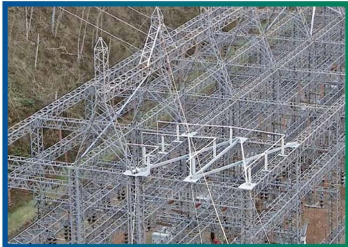
**SOUTHWESTERN AND CORPS PERSONNEL DESIGNED A SOLUTION USING AN OVERHEAD TRANSMISSION LINE FROM THE SWITCHYARD TO RETURN UNIT 1 TO SERVICE.**
