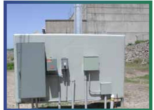
**A NEWLY INSTALLED EQUIPMENT BOARD CONSOLIDATED JUNCTION BOXES, POWER PANELS, AND OTHER EQUIPMENT AT BROKEN BOW.**
