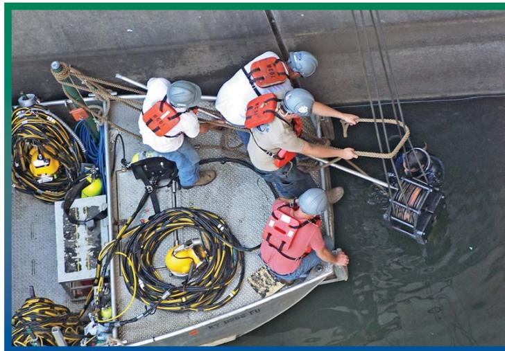
**UNDER A CORPS CONTRACT FUNDED BY ARRA, DIVERS SUCCESSFULLY RETRIEVE A BROKEN BLADE THROUGH THE DRAFT TUBE OPENING AT STOCKTON DAM IN AUGUST 2009, THE FIRST MILESTONE EVENT IN THAT PROJECT'S REHABILITATION.**
