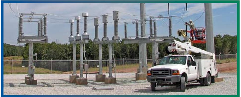
**GORE SUBSTATION CREW ELECTRICIAN JIM O'KELLEY TESTS LIGHTNING ARRESTERS TO INSURE THEY PERFORM AS DESIGNED.**
