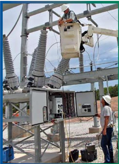
**WORKING FOREMAN TONY COCHRAN (IN BUCKET) AND ELECTRICIAN ROBERT VAN BRUNT WORK CAREFULLY AROUND A GAS BREAKER TO PERFORM EQUIPMENT TESTS.**
