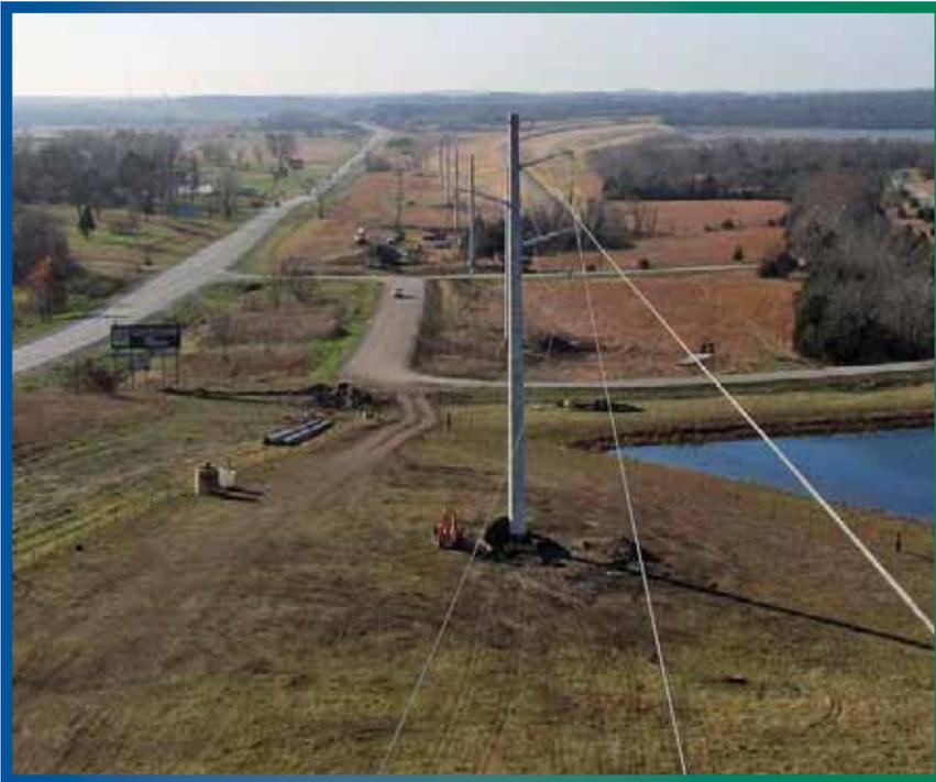
**SINGLE-POLE CONCRETE TRANSMISSION STRUCTURES WERE THE IDEAL SOLUTION FOR THIS LINE RELOCATION UNDERTAKEN TO ACCOMMODATE THE FUTURE WIDENING OF U.S. HIGHWAY 65 NEAR TRUMAN LAKE IN CENTRAL MISSOURI.**
