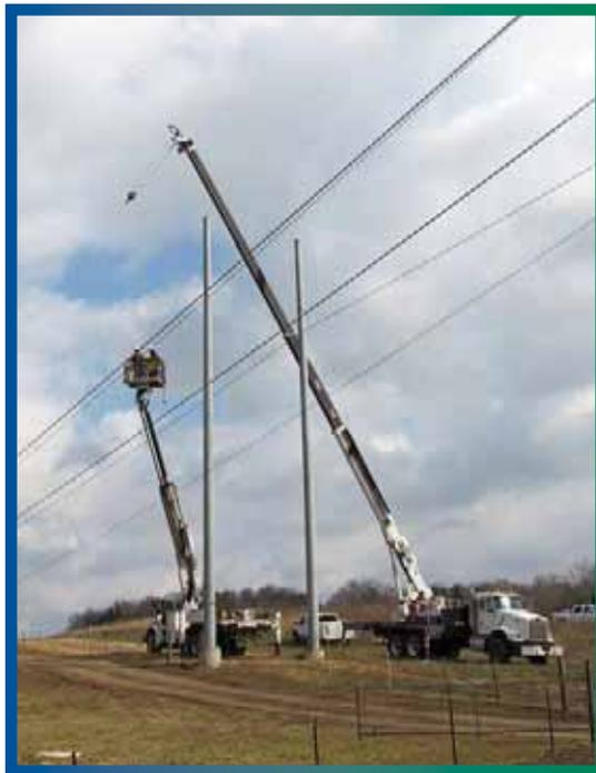
**THE SPRINGFIELD LINE CREW MOVES CONDUCTOR FROM A STEEL H-FRAME STRUCTURE ON SOUTHWESTERN'S LINE 3025 NEAR TRUMAN LAKE AS PART OF A RELOCATION THAT INVOLVED THE COOPERATION OF THE MISSOURI DEPARTMENT OF TRANSPORTATION, THE CORPS, AND SOUTHWESTERN.**
