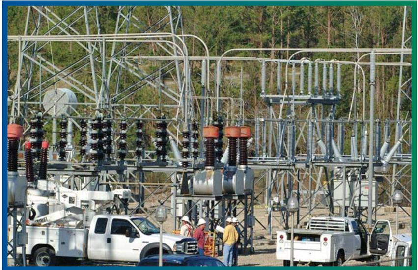
**NEW RENOVATIONS ARE DISTINGUISHED IN THIS PHOTO BY THE COLOR OF INSULATOR. THE NEWER GRAY INSULATORS ON THE RIGHT CONTRAST WITH THE BROWN INSULATORS OF THE OLDER EQUIPMENT.**
