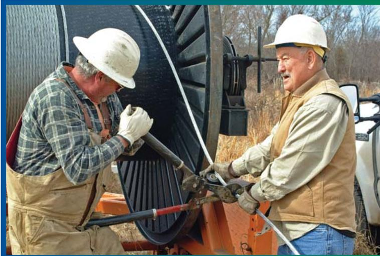
**TOP: LINE EQUIPMENT OPERATOR MICHAEL KOENIG AND LINEMAN GARY GREGORY CUT A SECTION OF FIBER AT THE EXPLORER TAP TO COMPLETE THE OPTICAL GROUNDWIRE AND MICROWAVE COMMUNICATIONS SYSTEM STARTED 11 YEARS AGO.**
