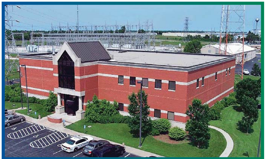
SOUTHWESTERN'S SPRINGFIELD OPERATIONS CENTER BUILDING, CONSTRUCTED IN 1996, AND THE REMODELED MAINTENANCE BUILDING BEHIND IT, INCORPORATE MANY OF THE ENERGY EFFICIENT STANDARDS AND SUSTAINABLE PRACTICES REQUIRED FOR GOVERNMENT FACILITIES BY EXECUTIVE ORDER 13423.
