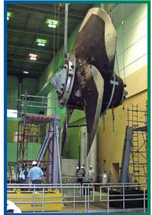
**ABOVE: THE OLD RUNNER HUB IS REMOVED FROM UNIT #4 FOR REPLACEMENT AS PART OF A MAJOR REHABILITATION THAT WILL INVOLVE ALL FIVE TURBINES AT OZARK DAM POWERHOUSE.**
